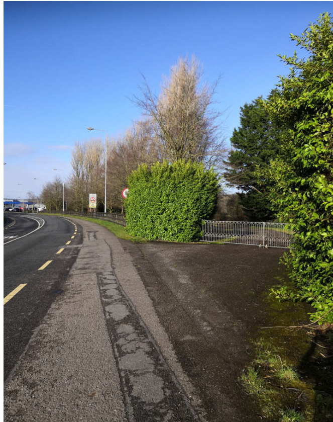
Figure A.3: Existing weigh-station gate to south of proposed entrance junction
