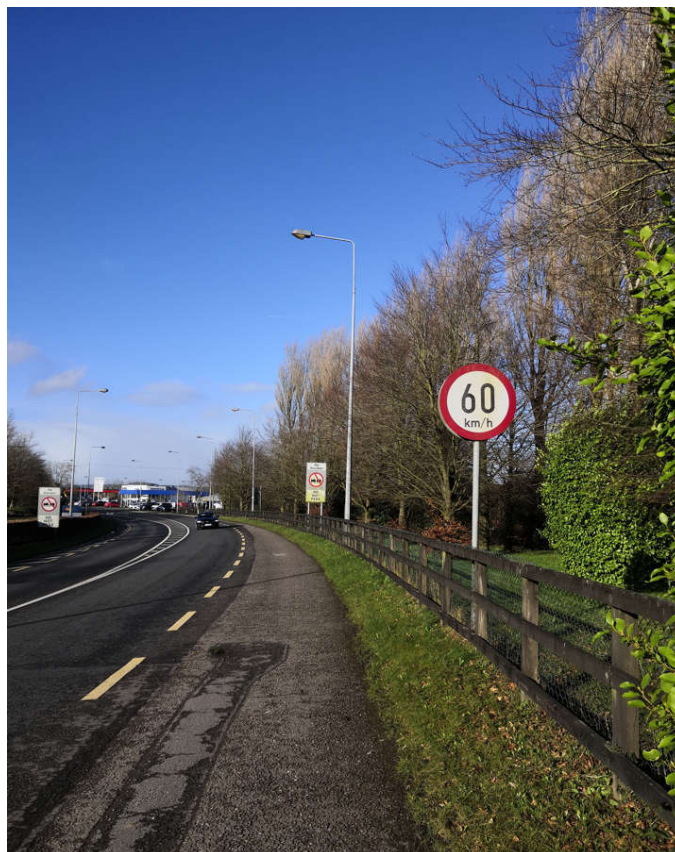
Figure A.4: Location of 60 kph signpost located to the south of the proposed entrance junction
